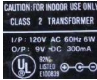
Close up of the transformer label.
